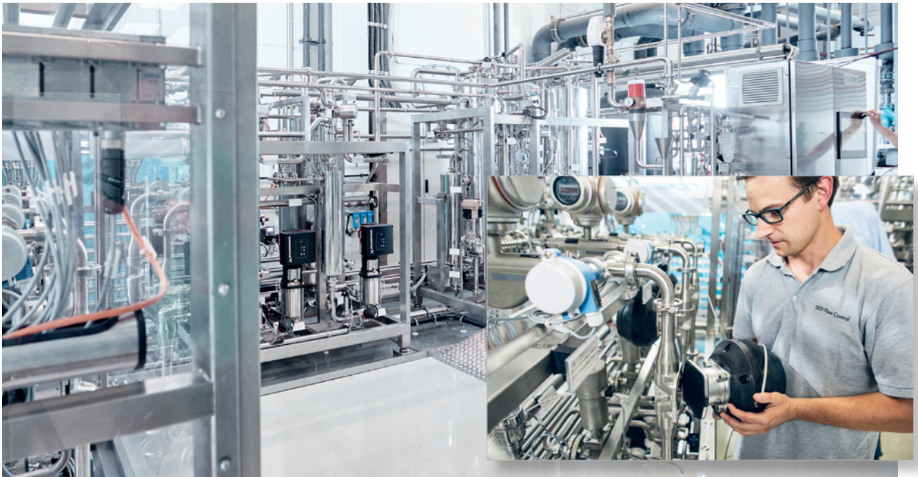
Process test bench. Cycle and lifetime testing of diaphragms and valves with saturated steam and various cip media.
