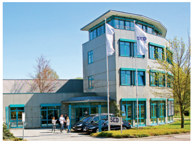
The office building is connected to the production building for direct communication with manufacturing.
